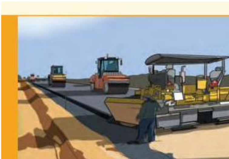
Picture 3: Road construction work
